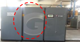
Installation of new receiver and new air compressors (not inverter type)
