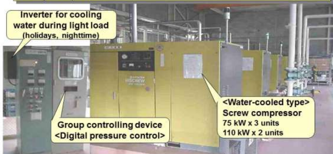
Outline of water-cooled air compressor (before renewal)
