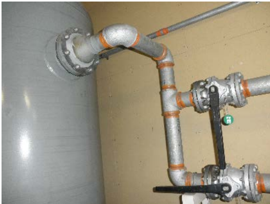
Large-bore pipe and receiver tank with adequate capacity
