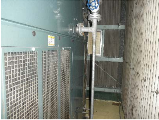
Provide a drain plug for a riser pipe.
