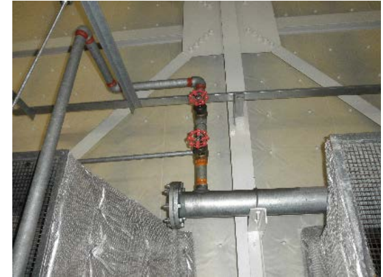
Riser pipe installed from above
