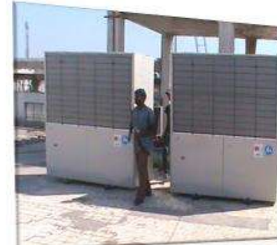
Gas heat pump (outdoor unit)
