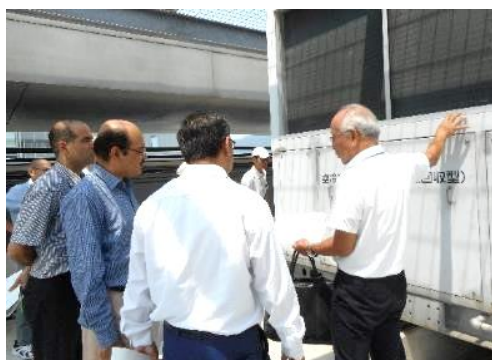
Visit to EHP facility (manufactured by Mayekawa MFG. Co., Ltd.) installed at Hyogo Prefectural Museum of Art
