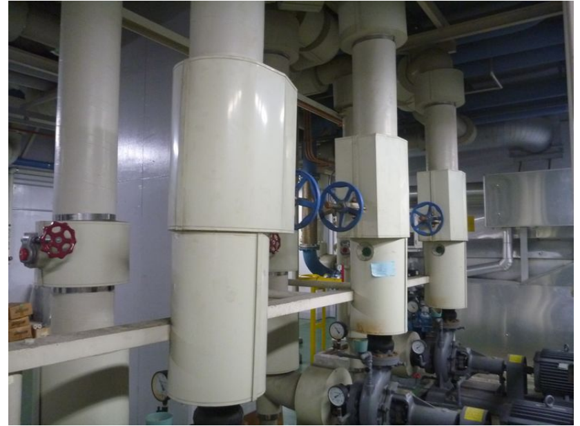
Hot water: with insulating cover
