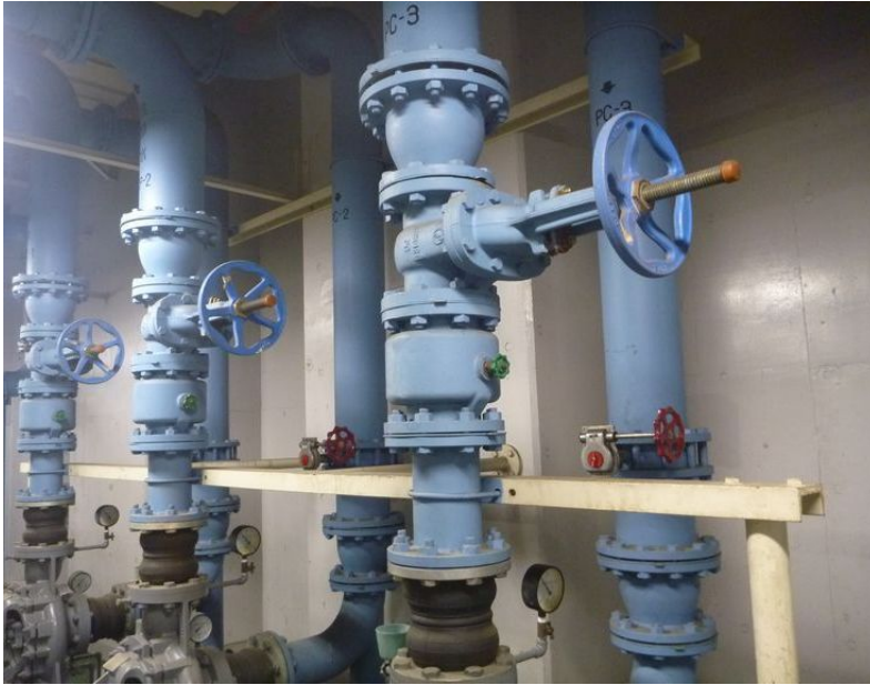
Cold water: w/o insulating cover
