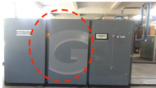
Installation of new receiver and new air compressors (not inverter type)
