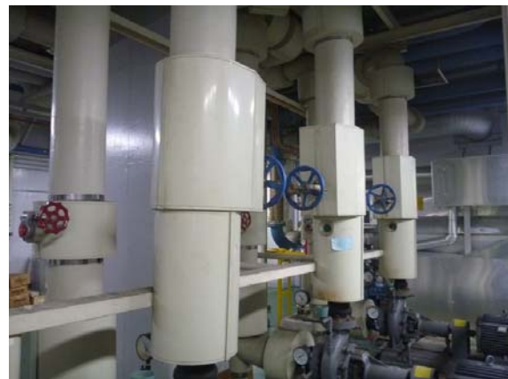
Hot water: with insulating cover
