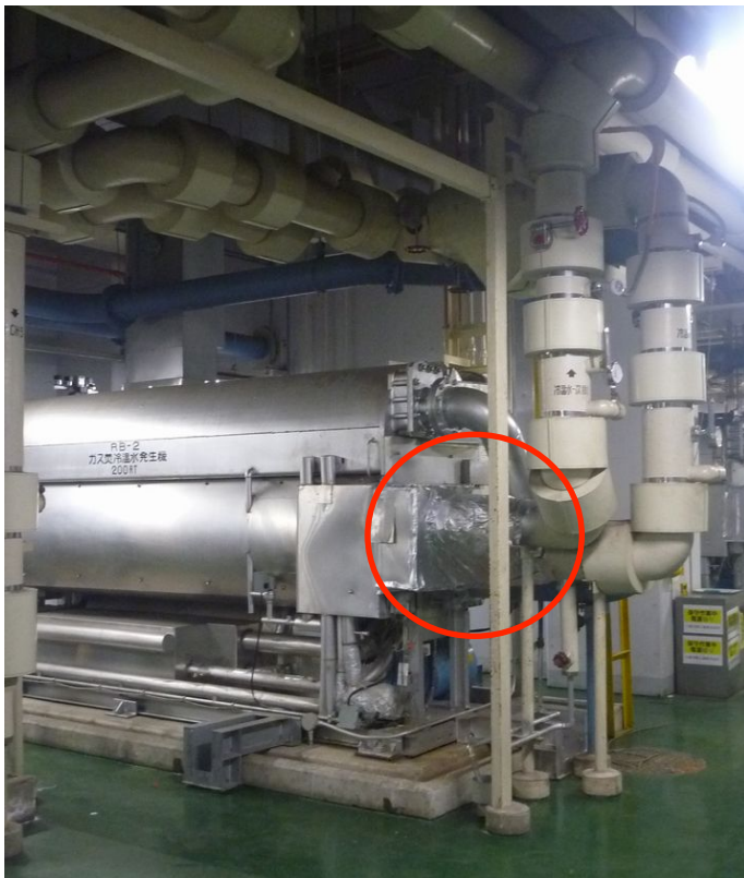
Cold/hot water generator for air conditioning
