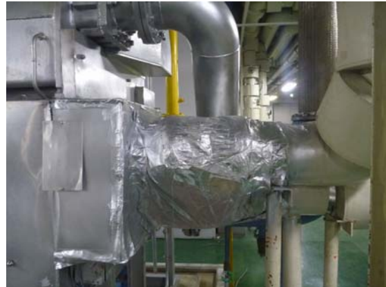
Heat retaining by insulating cover
