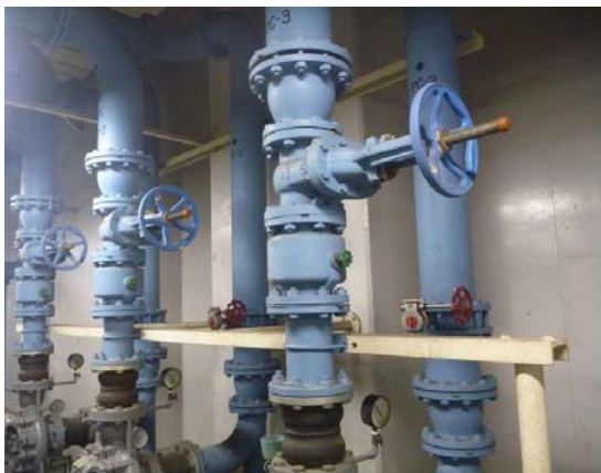
Cold water: w/o insulating cover
