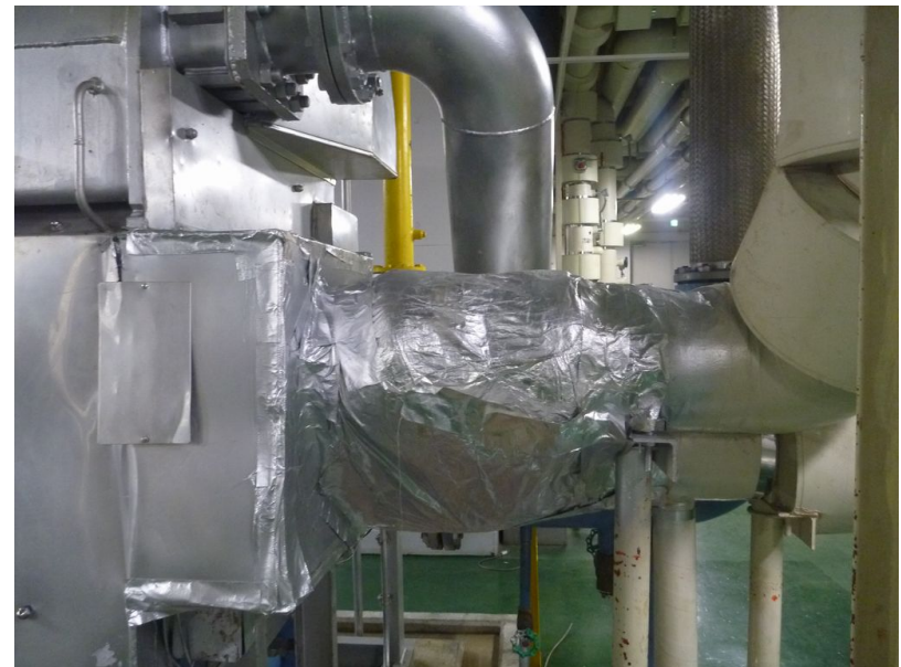
Heat retaining by insulating cover
