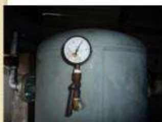
(4) Check the pressure sensor mounting position (air receiver tank pressure gauge). * A place where instant pressure fluctuation is small.
