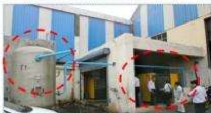
e.g.1: Installation of new receiver and new air compressors (not inverter type)
