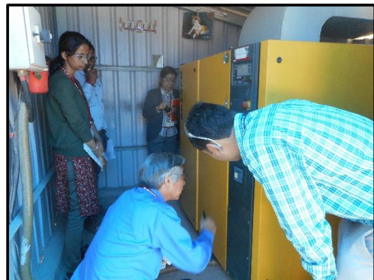
Site visit, Gopal Glass Works
