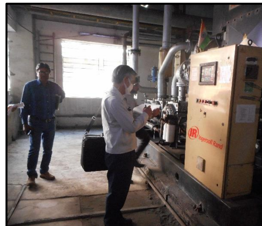
Site visit, Jindal Worldwide Ltd
